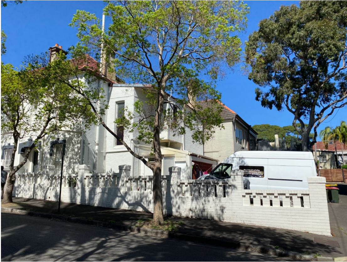
Allen Street (Avenue Lane to right)
